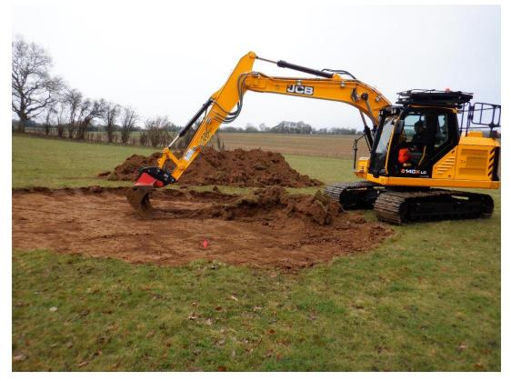
Plate 2. Topsoil strip (looking South)
